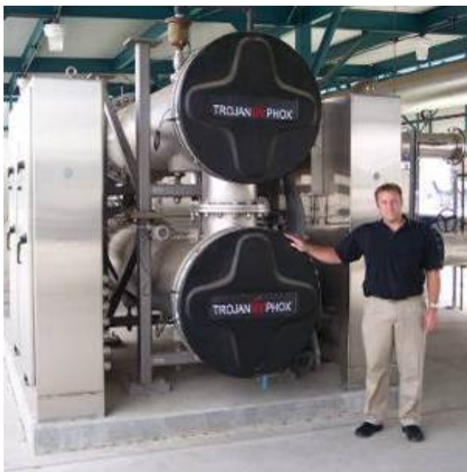
Figure 1 UV/Hydrogen Peroxide Treatment System, Trojan Technologies UVPhox
