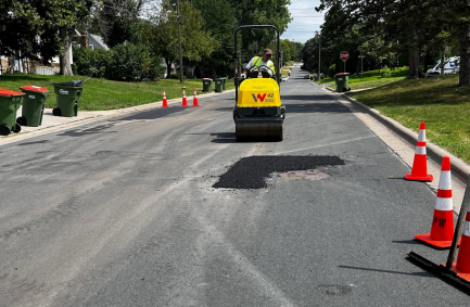
73 tons of asphalt to repair pavement
